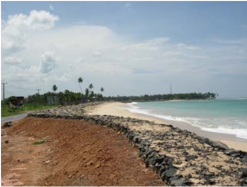
Bank Revetment; Sri Lanka
