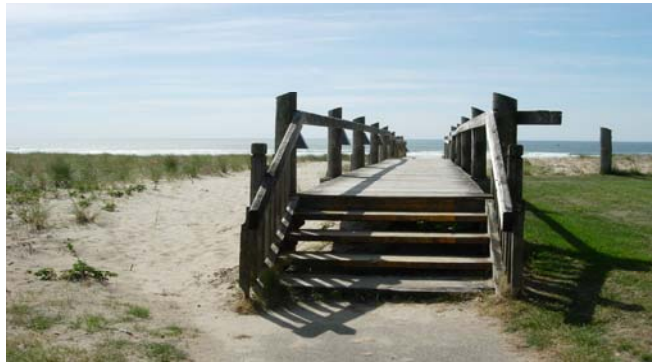
Structure pathway for particularly sensitive dune (Oregon, USA)
