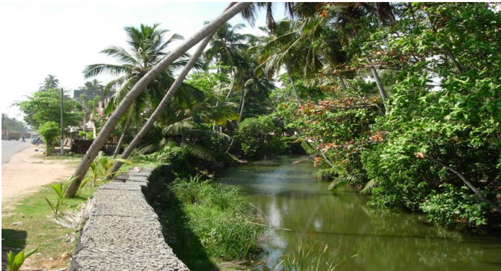
Retaining wall to stabilize roadway: Marissa, Sri Lanka
