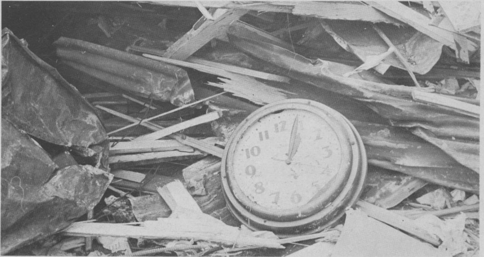
The clocks stopped—and so did nearly everything else in Hilo—when the wave struck shortly after 1 a.m., Monday, May 23, 1960.
