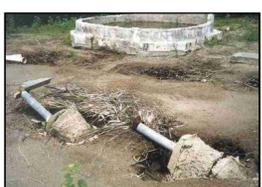
All that remained of Sissano Government Station office building were the foundations and part of a concrete water tank.
