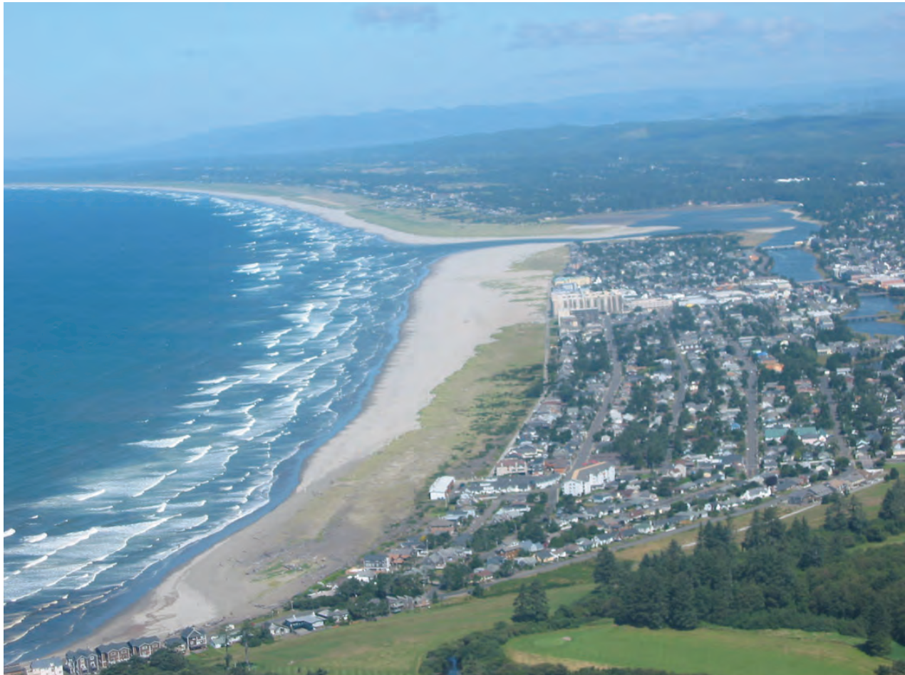
Figure 2: Oblique aerial view looking from the south toward Seaside, Oregon, shown in the foreground. The mouth of the Necanicum River separates Seaside from Gearhart in the distance (courtesy of the United States National Agriculture Imagery Program (NAIP)).
